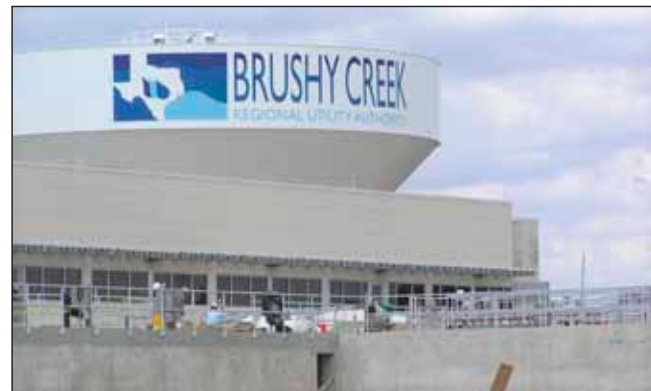
The Brushy Creek Wastewater Treatment Plant
